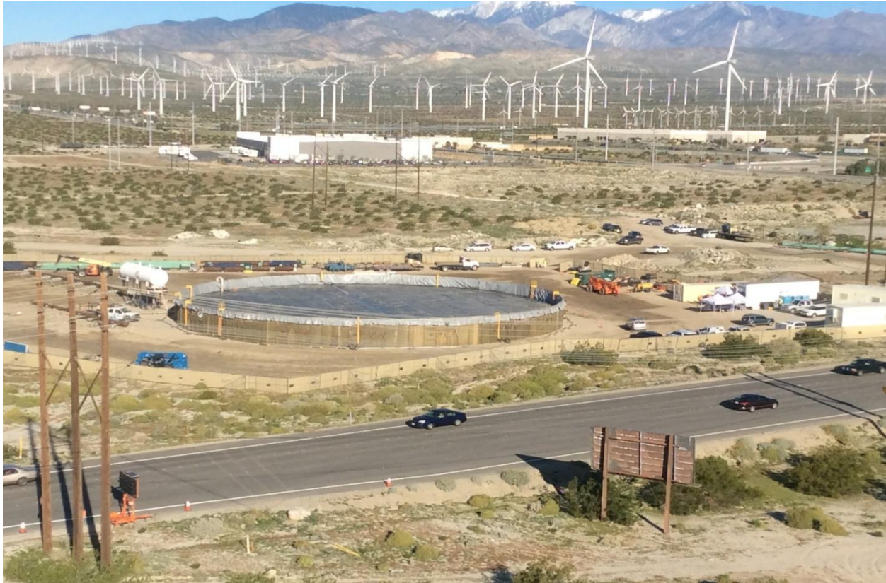
Figure 10: Temporary Lake Tank to Store Water for Hydrotest
