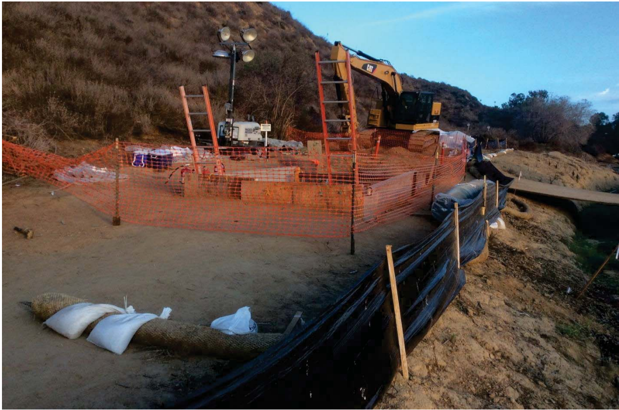
Figure 24: Section 4 and 5 West End Test Head Excavation
