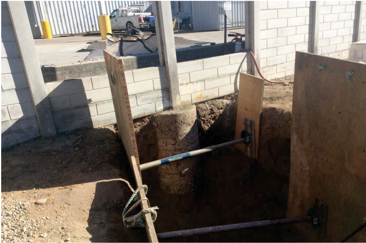
Figure 16: Section 1 Existing Wall Footing Within Trench
