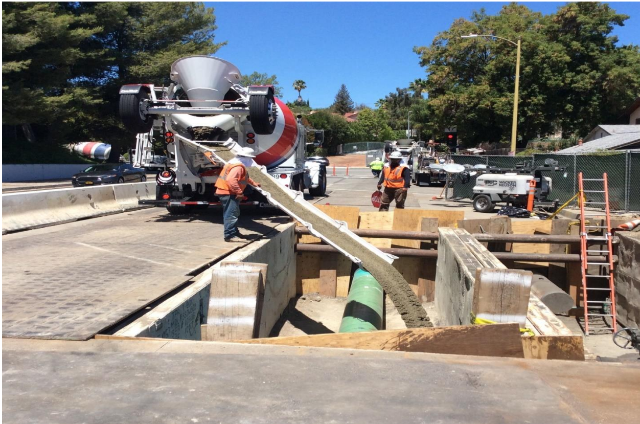
Figure 10: Backfilling Bell Hole Line 406 at Burbank Boulevard
