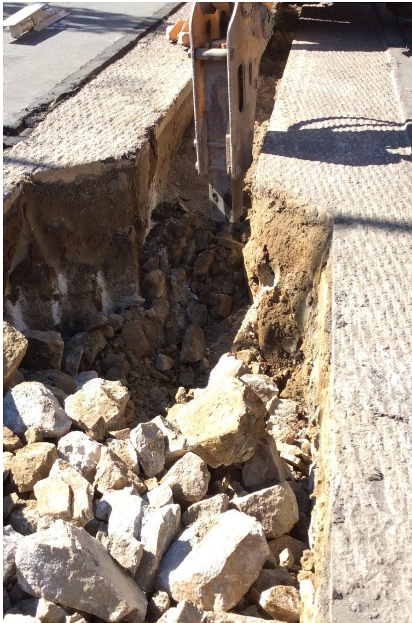
Figure 12: Breaking Rock (Granite)
