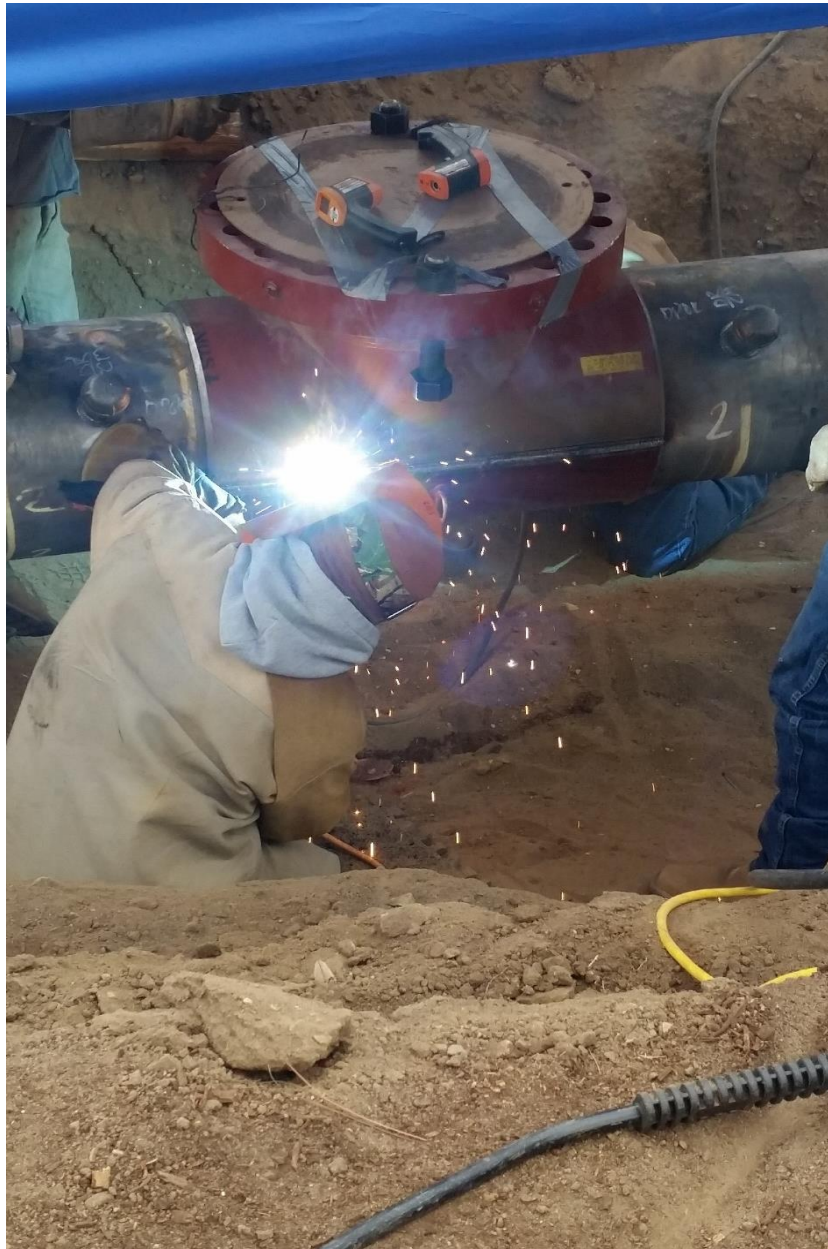
Figure 6: Welding of Stopple Fitting at Battles Road
