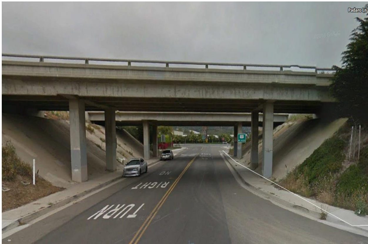
Figure 7: Underpass Site of New Crossover Line 8119
