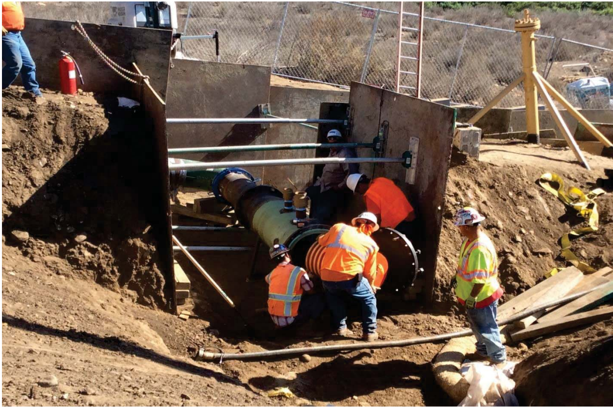
Figure 18: Section 2 Hydrotest Prep at Hall Canyon Site
