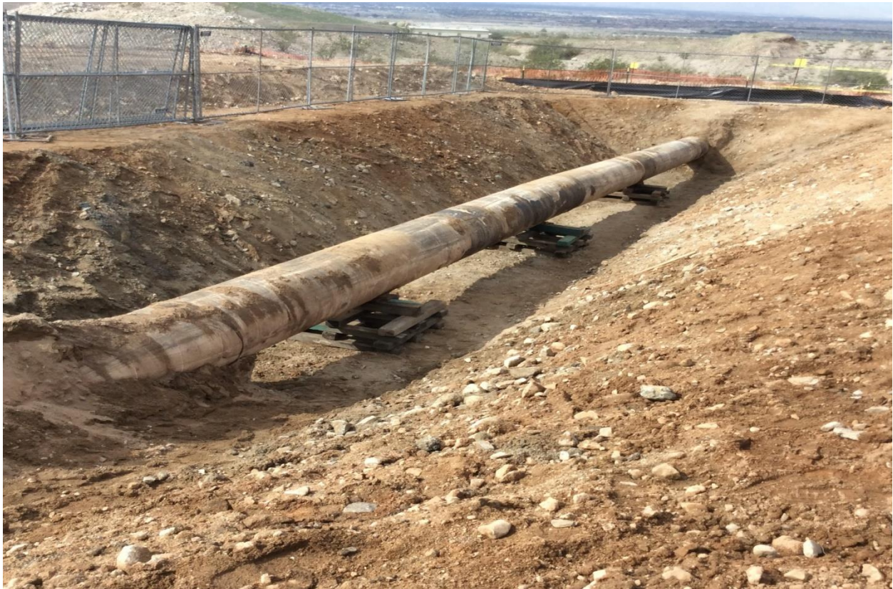
Figure 9: Temporary Pipe Supports (TB-7) Under Line 2000 in Preparation for a Test Break
