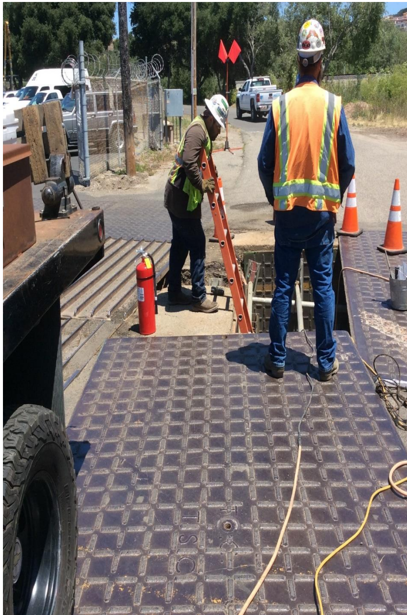
Figure 4: Setting up to Weld on Bello Street
