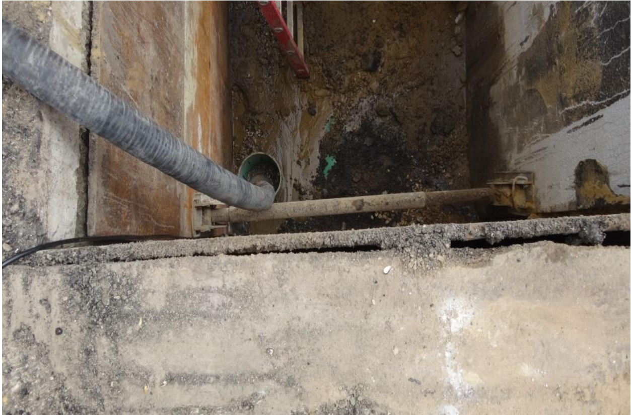
Figure 10: Groundwater Mitigation
