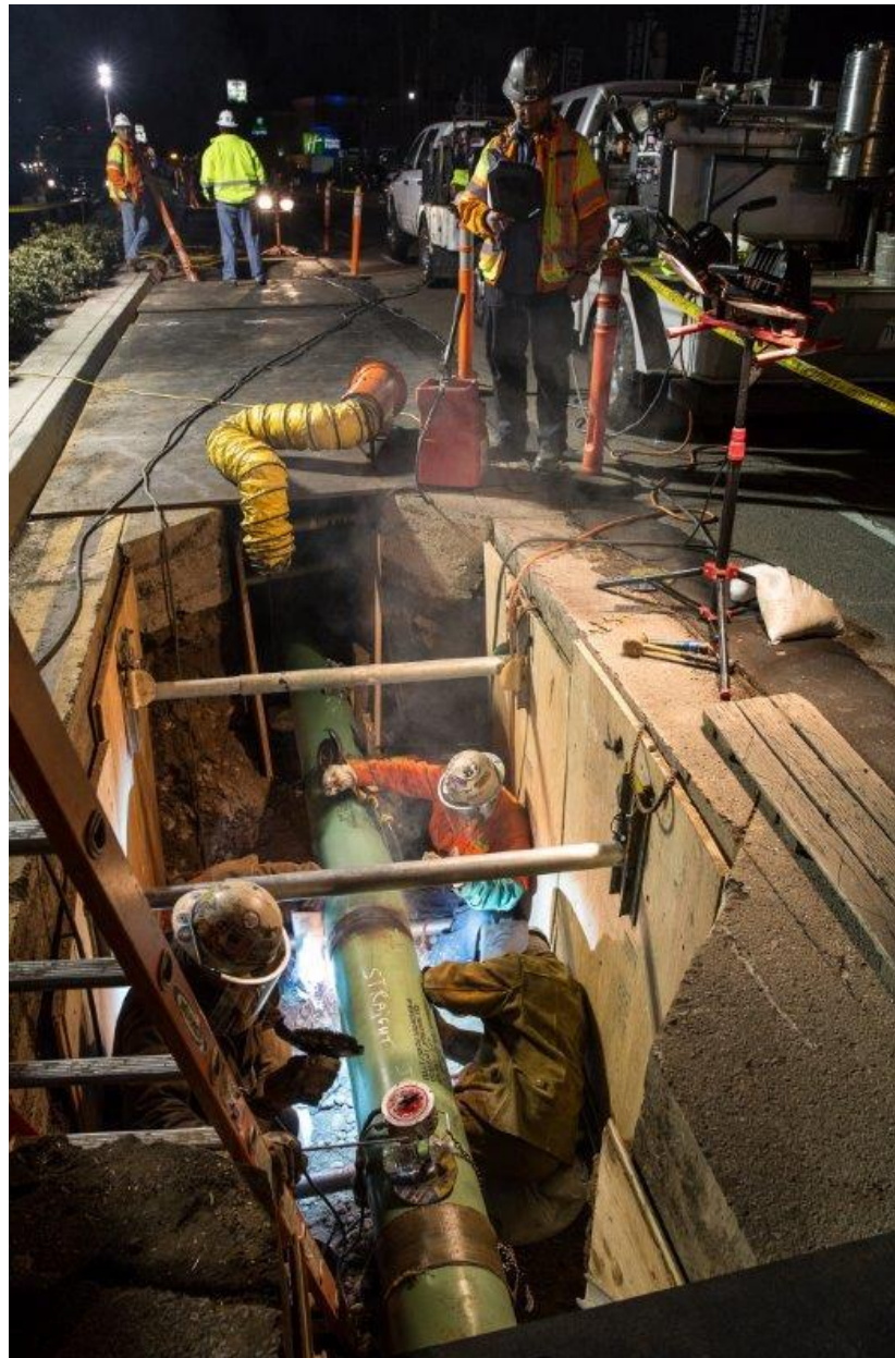
Figure 8: Night Work on Mission Bay Drive
