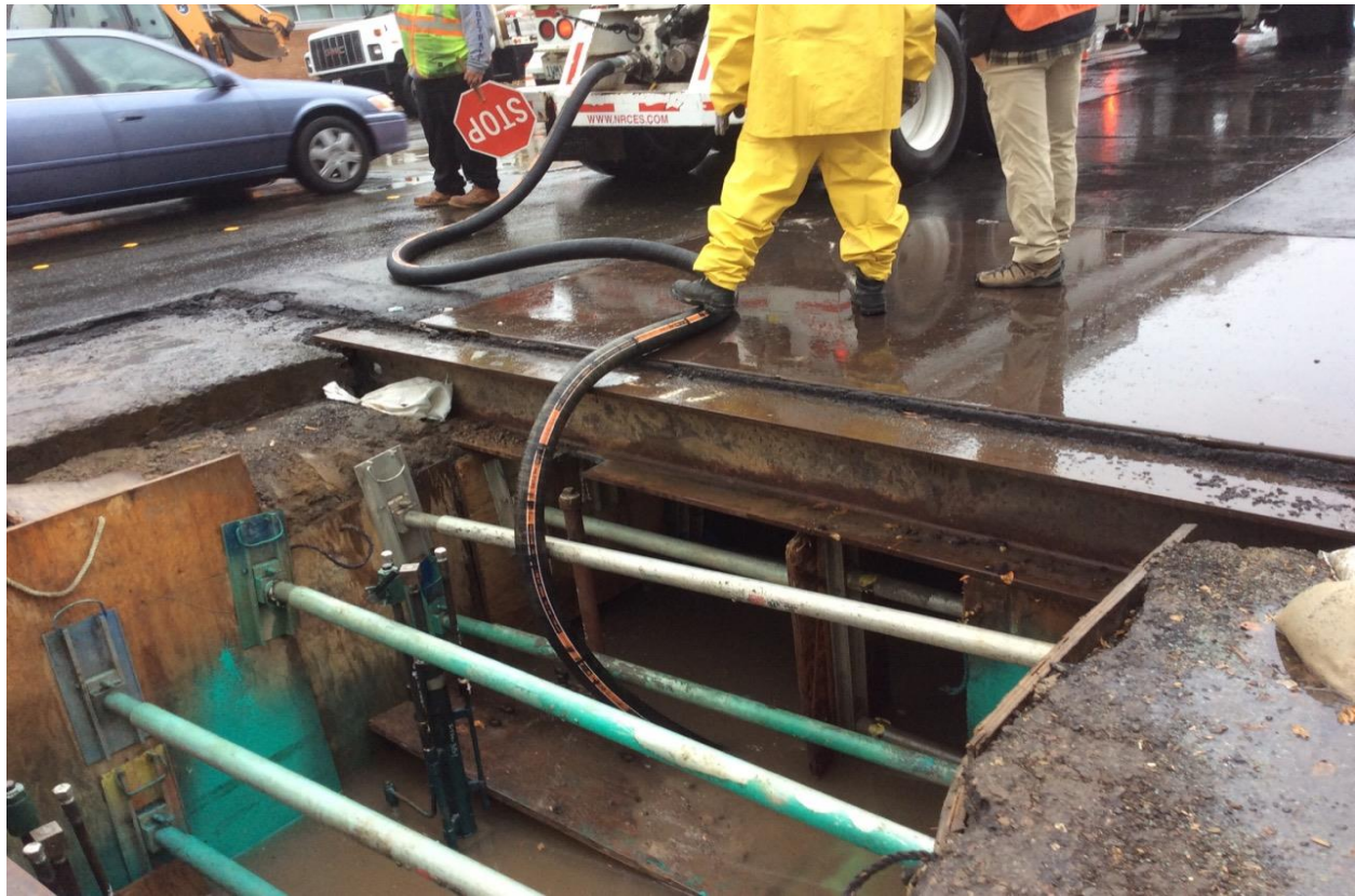
Figure 10: Pumping Water from Bellhole
