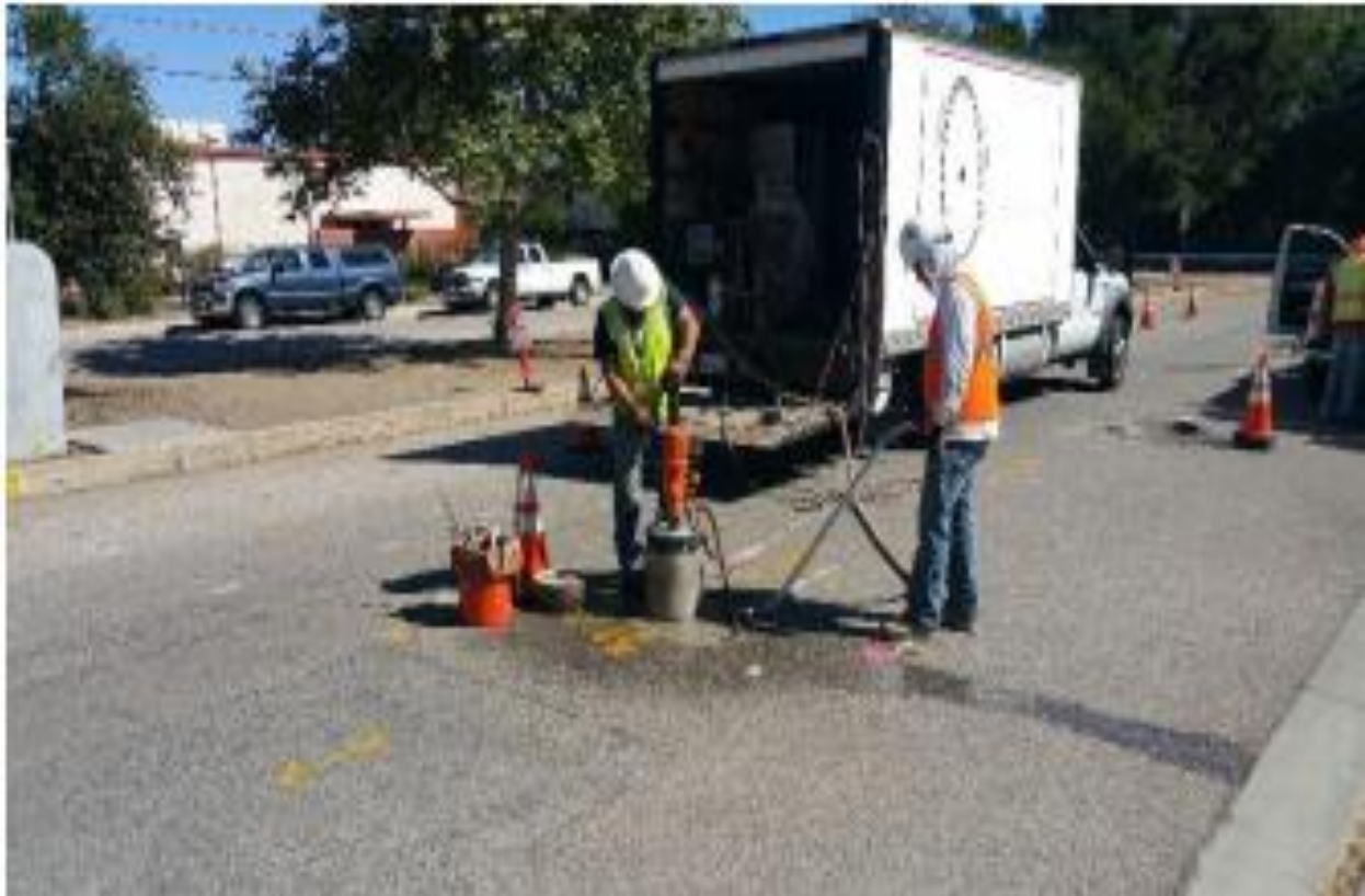
Figure 6: Potholing Operation
