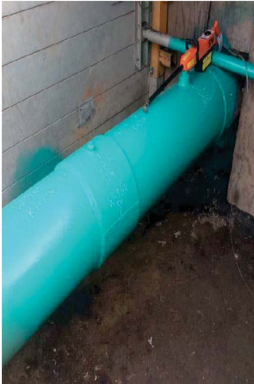
Figure 22: Section 3 Coating Inspection at Tie-in Point
