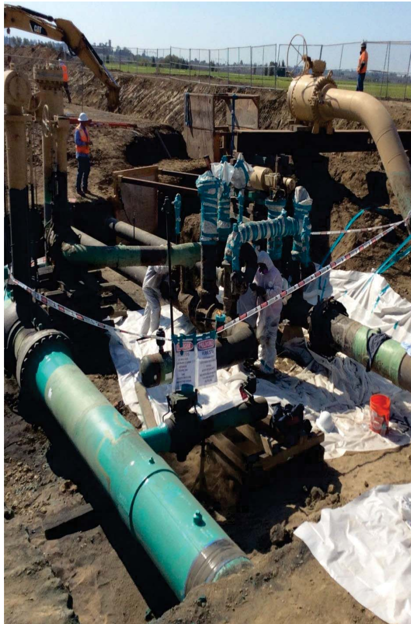
Figure 23: Section 3A Abatement Activities of MLV Removal
