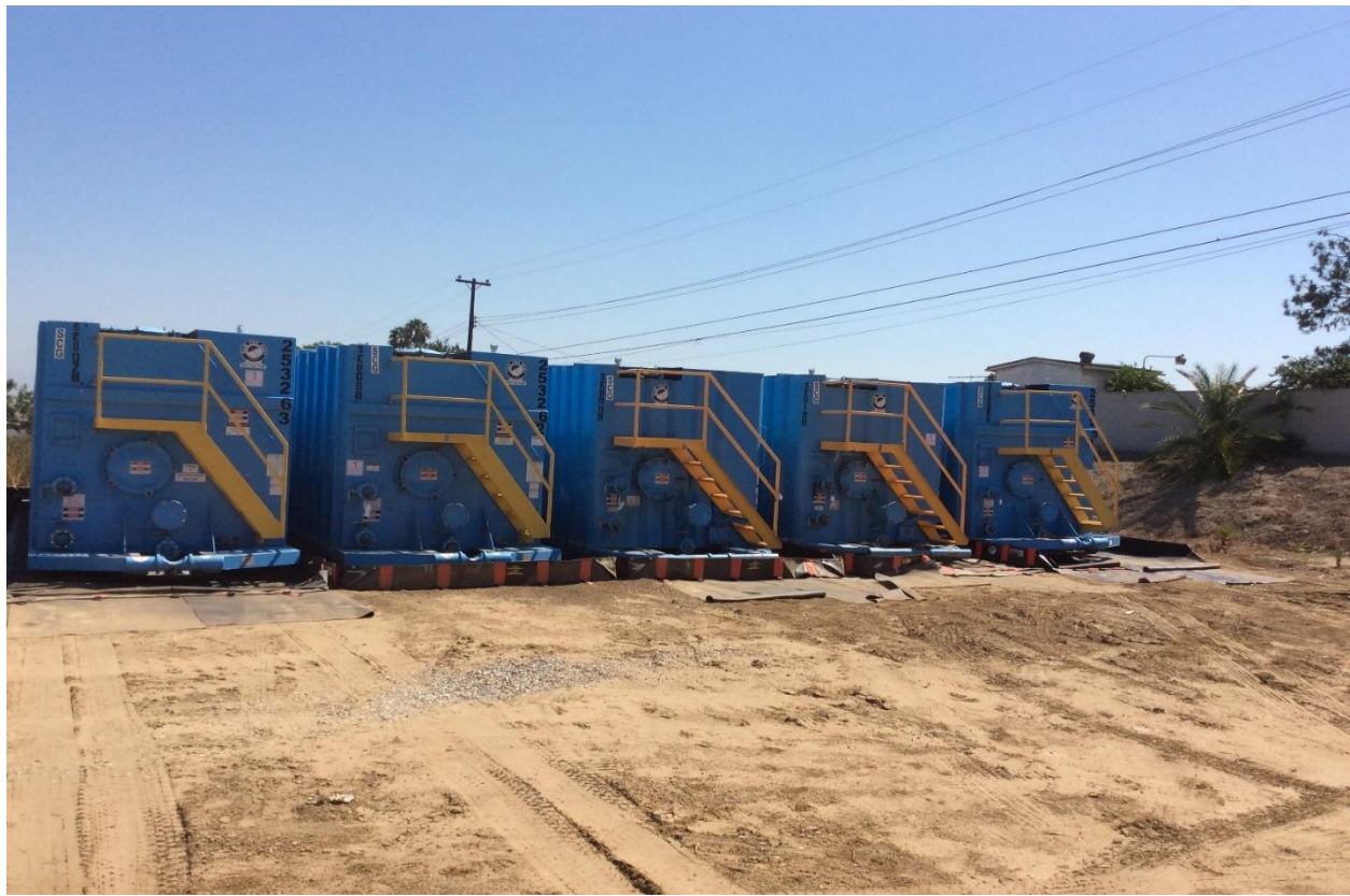
Figure 4: Water Storage Tanks for Hydrotest
