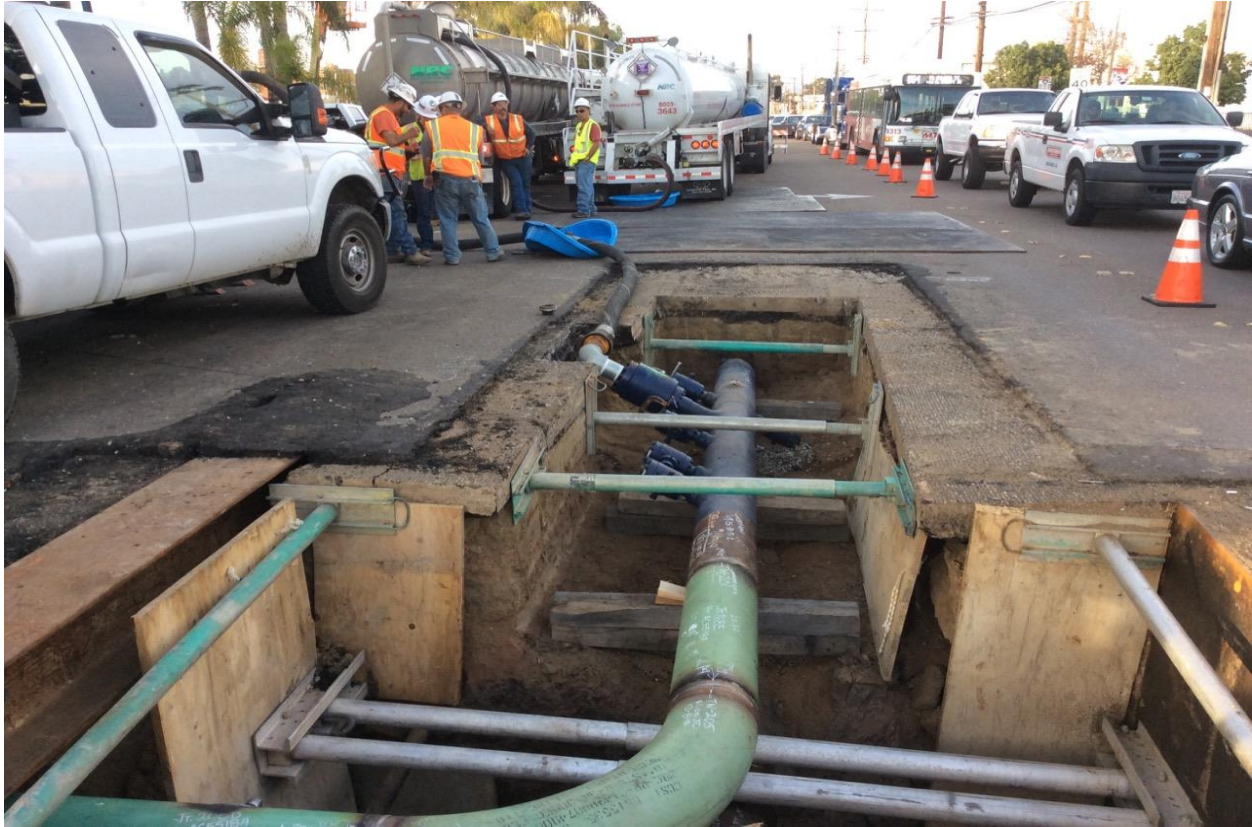
Figure 11: Hydrotest Contractor Setting Fill Pipe
