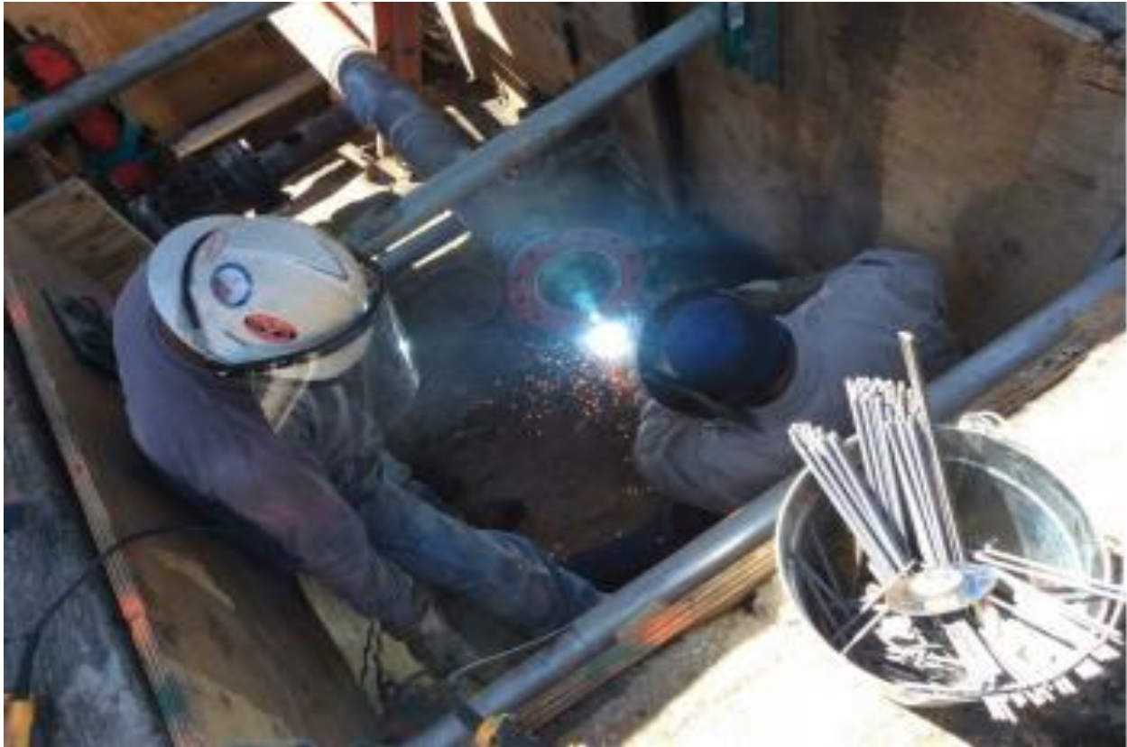
Figure 7: Installation of a Bottom Out Fitting
