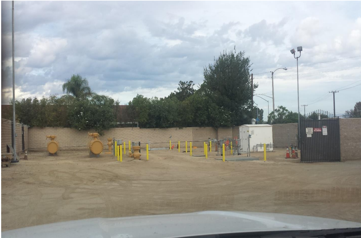
Figure 8: Station after Construction
