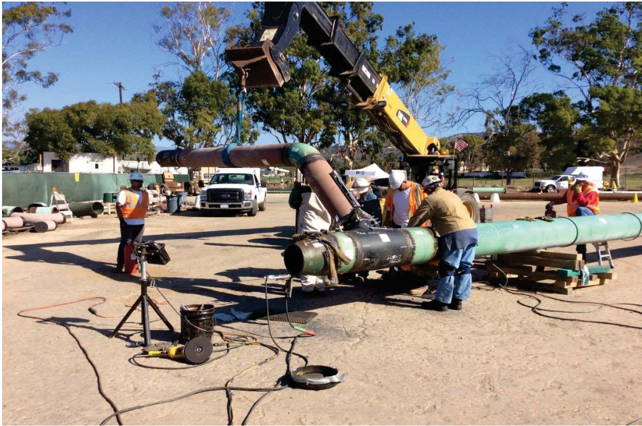
Figure 15: Section 1 Pre-fabrication of Replacement Pipe
