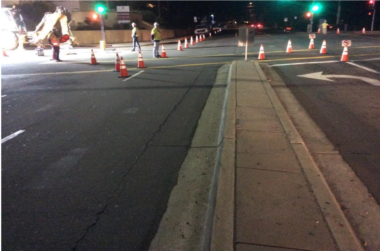
Figure 13: Traffic Control in Place
