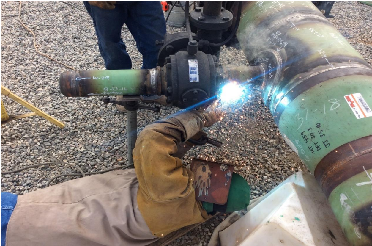
Figure 7: Fabrication of Bridle Tap and Valve on East Tie in Spool Added to Design
