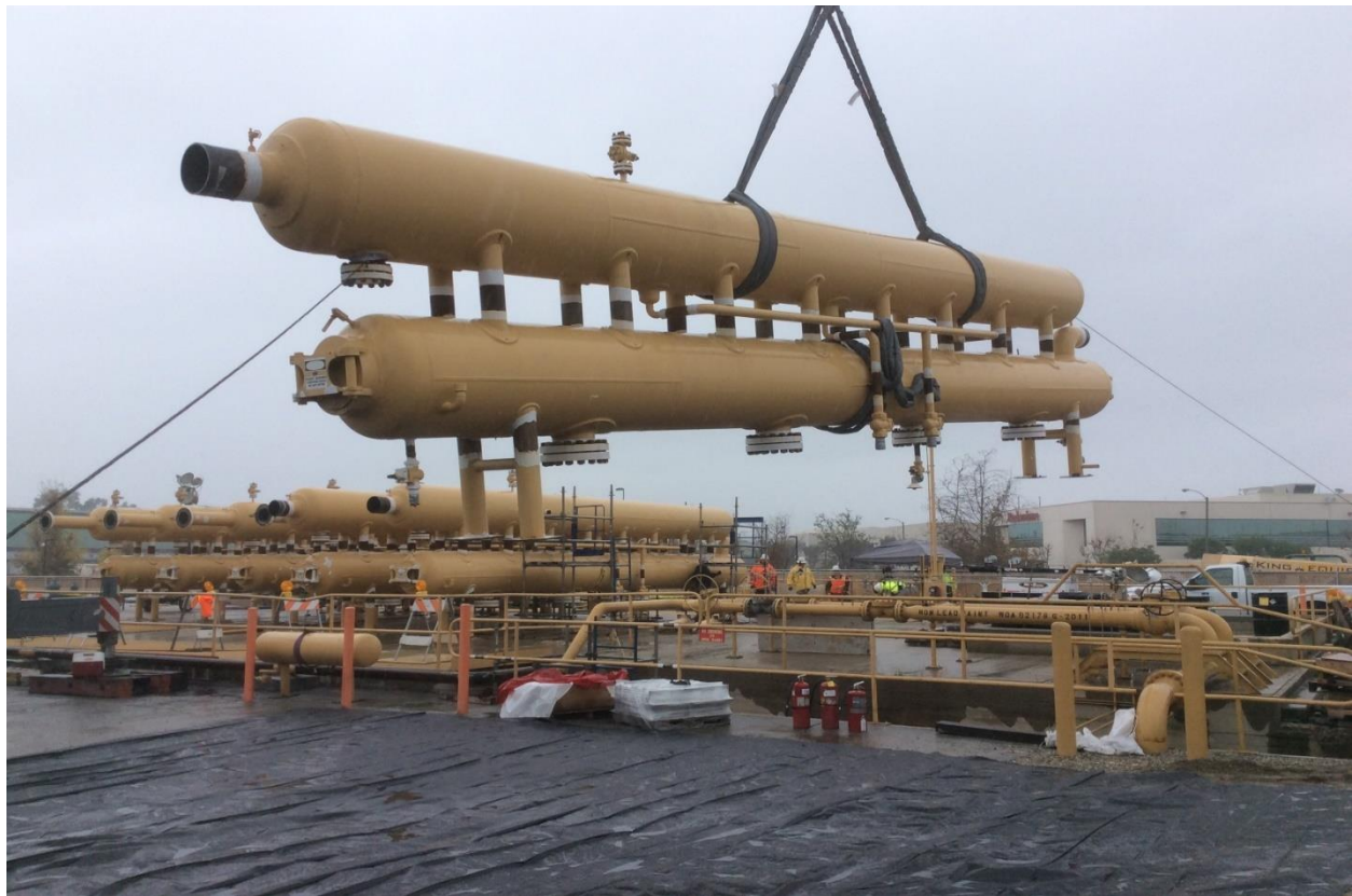
Figure 5: One (of Seven) Scrubber Assemblies Being Removed
