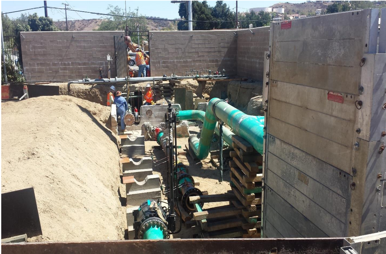
Figure 7: Construction within the Station
