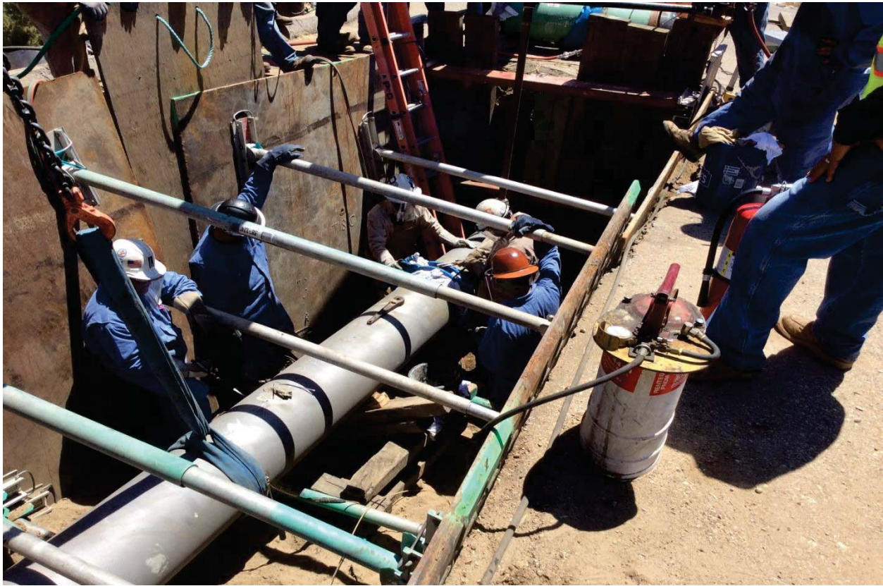
Figure 19: Section 2A Cut and Cap Activities
