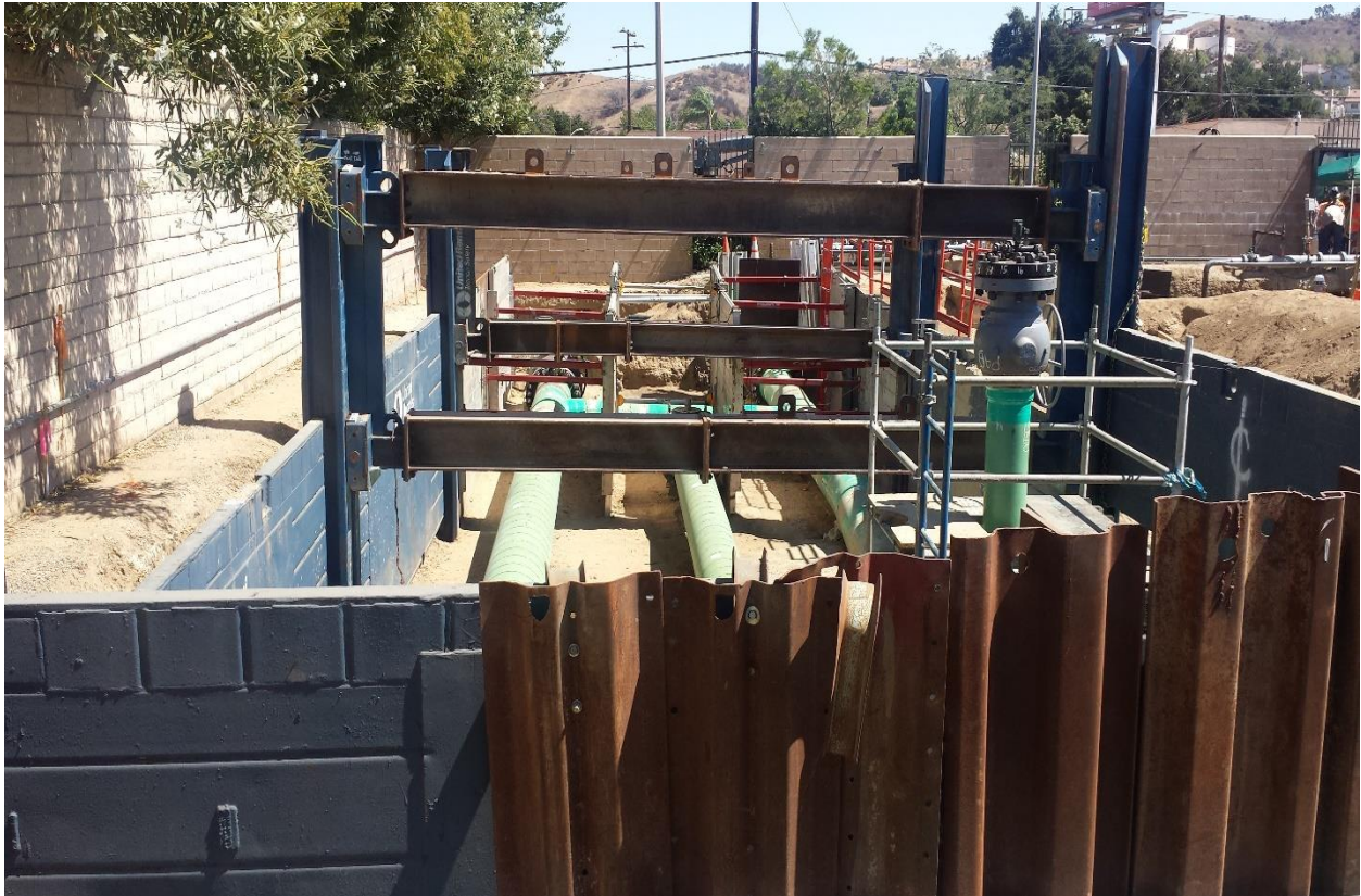
Figure 6: Shoring During Construction within Station
